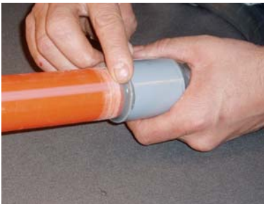
Smooth Excess Material
