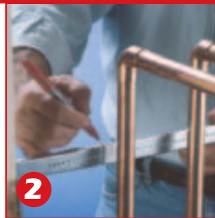
2 Position bracket and mark pipe locations
