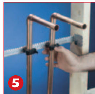
5 Secure the pipe by attaching TPC retainer
