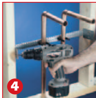
4 Install the TSGB to wall studs
