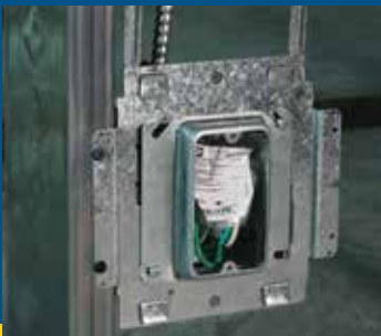
Time Savings on New Construction
