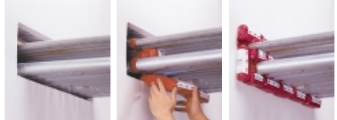
Conduit bank being firestopped.
