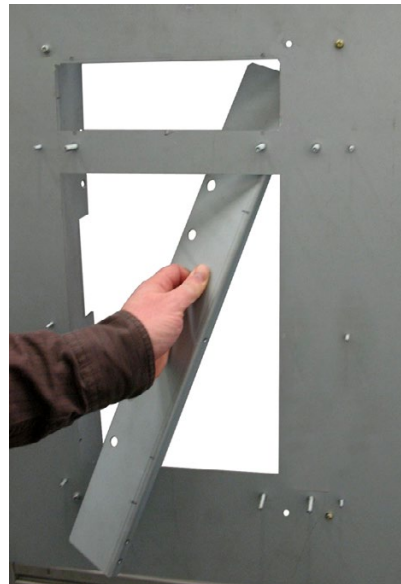
Insert the right reinforcement plate into the mounting cut-out.
